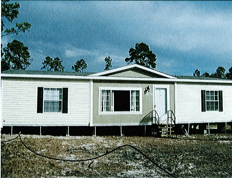
31 OCTOBER 2007 -- FRONT VIEW
