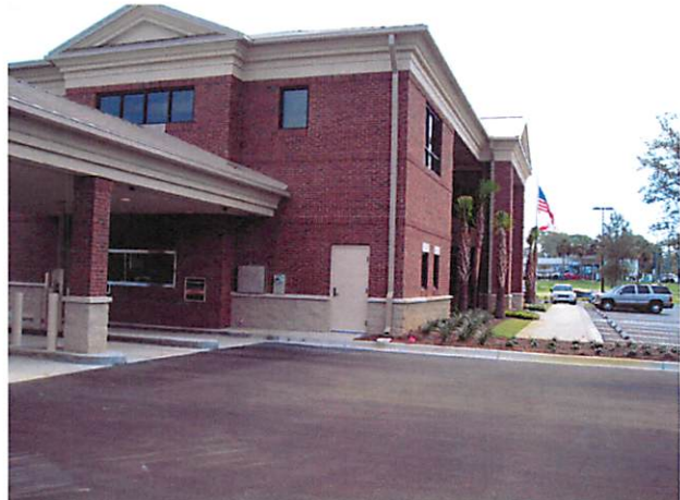
SIDE VIEW- WEST
