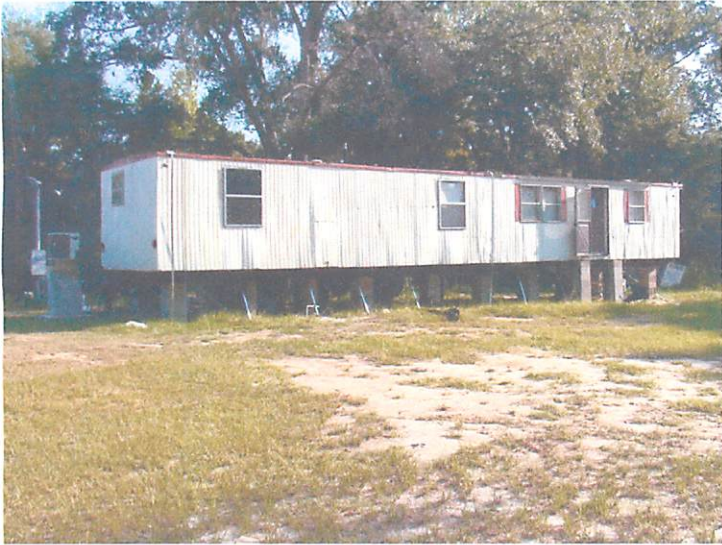
DATE: 8/30/2011 FRONT VIEW
