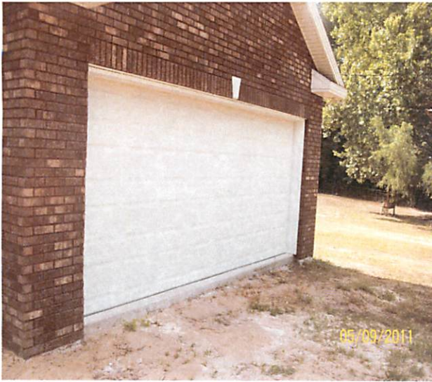
3134 B STREET - (FRONT) VIEW TAKEN 05-09-11
