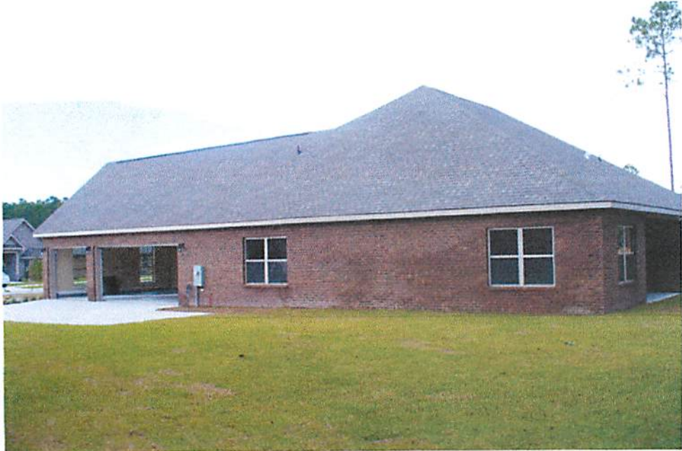
South (Right) Side view
