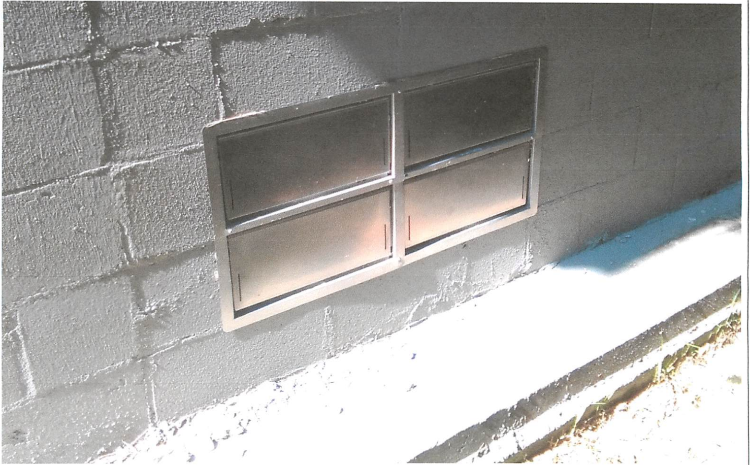
FLOOD VENTS LEFT SIDE VIEW 7/21/2015
