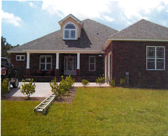
VIEW OF SOUTH SIDE OF HOUSE
