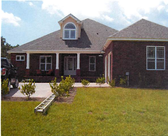
VIEW OF SOUTH SIDE OF HOUSE
