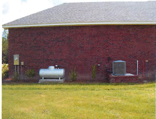
VIEW OF NORTH SIDE OF HOUSE
