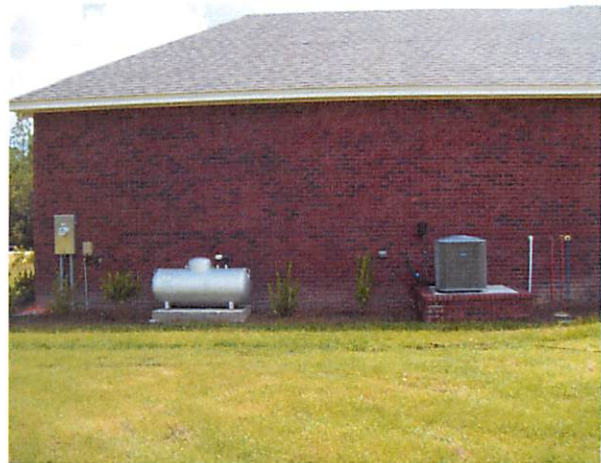
VIEW OF NORTH SIDE OF HOUSE
