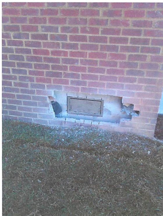
Garage Vents on Left Side of Garage - 3/31/2014
