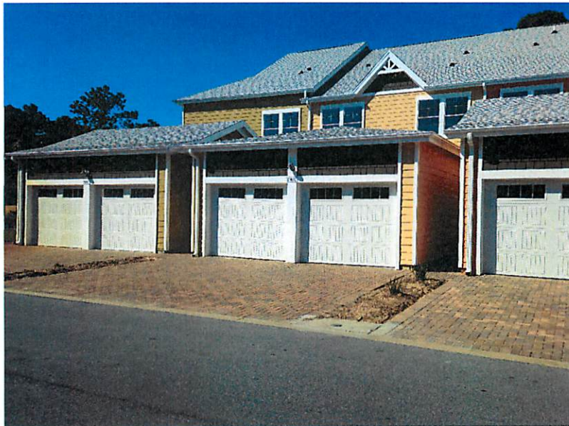
Rear View Photo Taken 10/20/14
