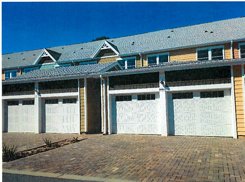
Rear View Photo Taken 10/20/14
