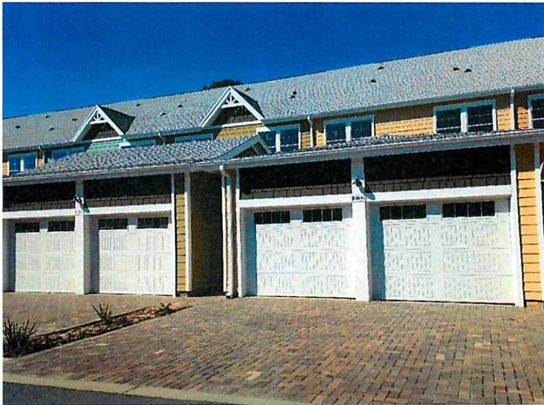
Rear View Photo Taken 10/20/14
