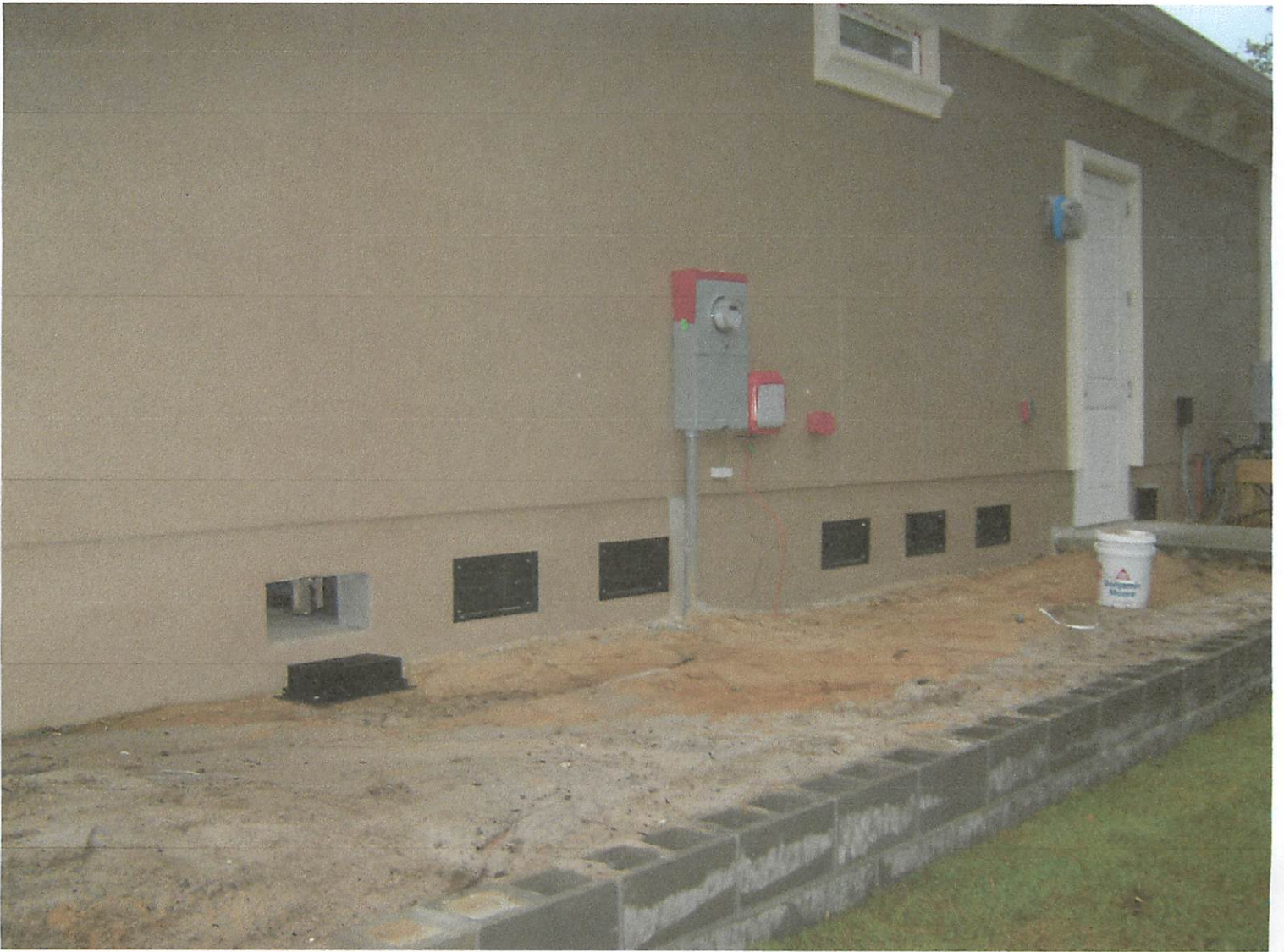
RIGHT SIDE VIEW-FLOOD VENTS
