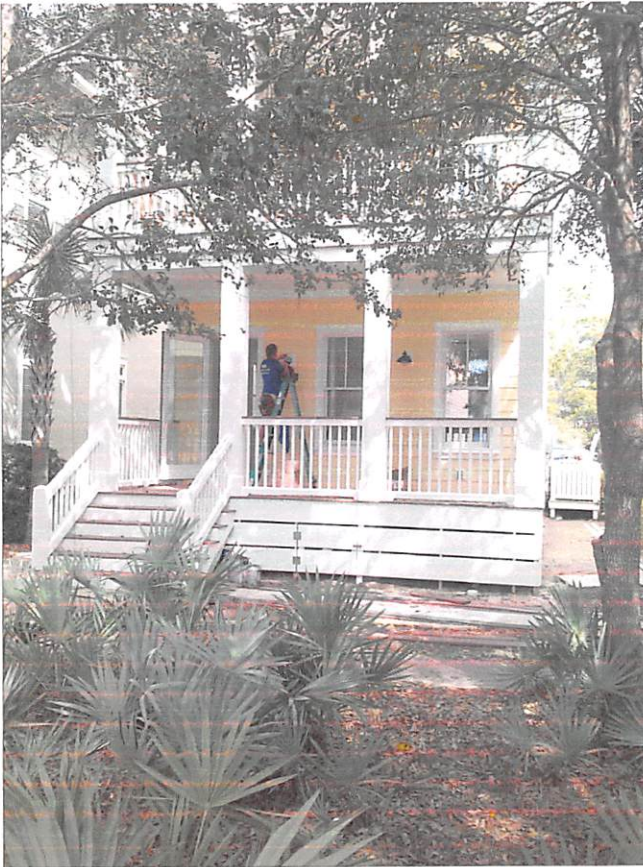
REAR VIEW – 03/10/2016 SOUTH SIDE
