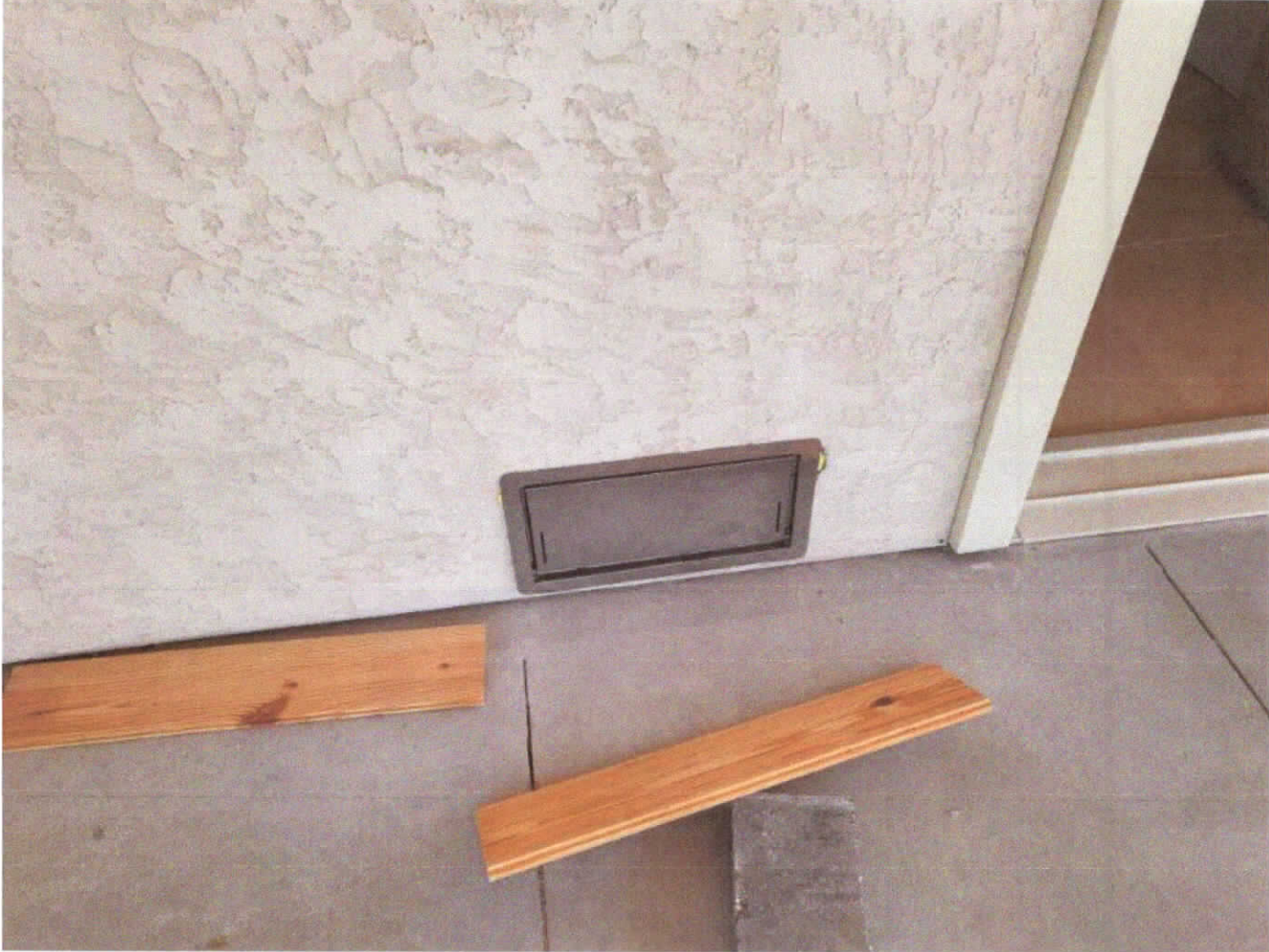
SMART VENT FLOOD VENT NORTH SIDE 10-13-2022
