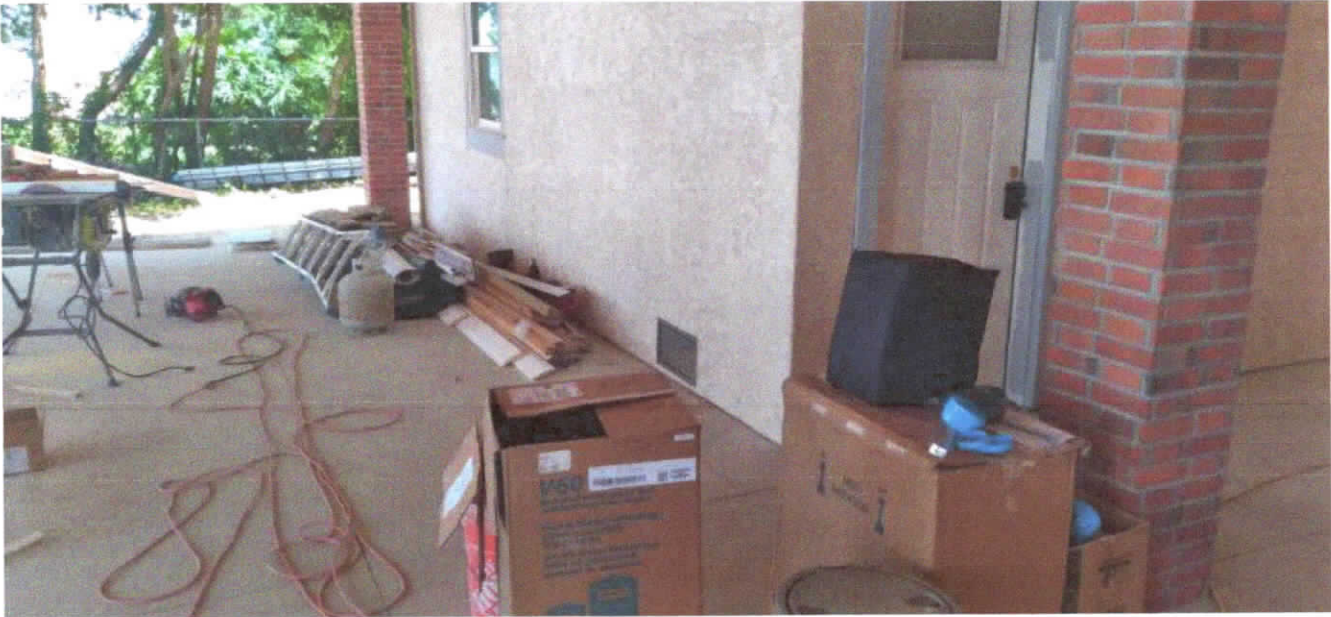
SMART VENT FLOOD VENT NORTH SIDE 08-19-2022
