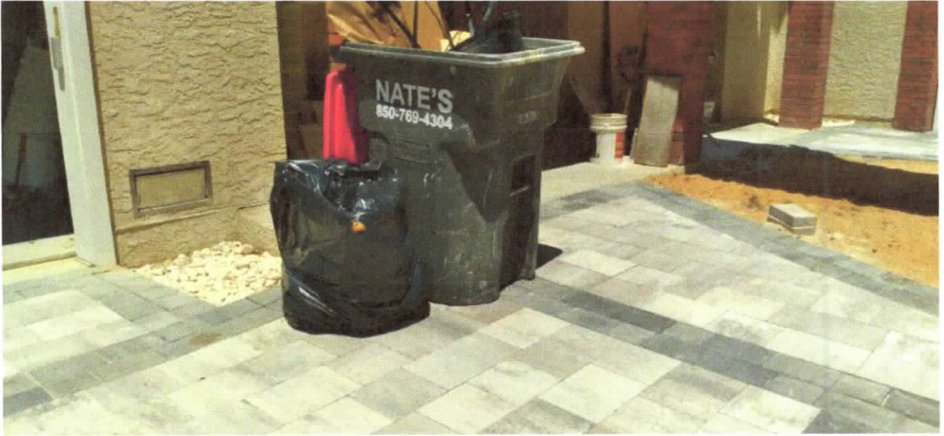
SMART VENT FLOOD VENT SOUTH SIDE 08-19-2022
