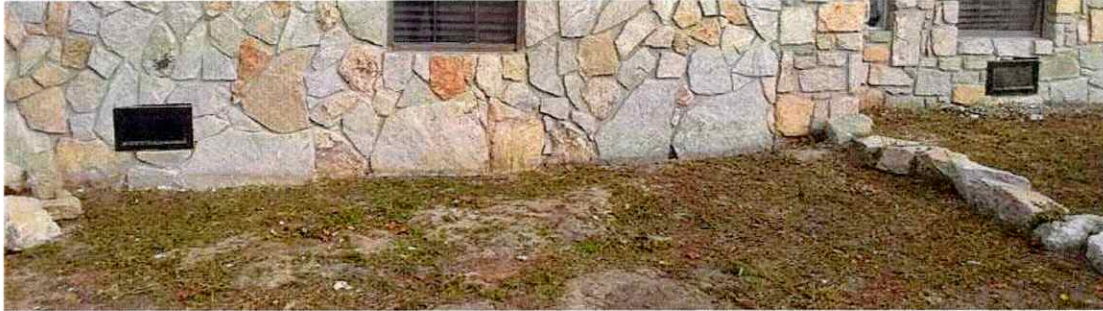
VENT 2 – 0.9' ABOVE GRADE 0.9' ABOVE GARAGE SLAB
