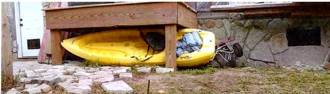
VENT 6 – 1.2' ABOVE GRADE 1.0' ABOVE GARAGE SLAB
