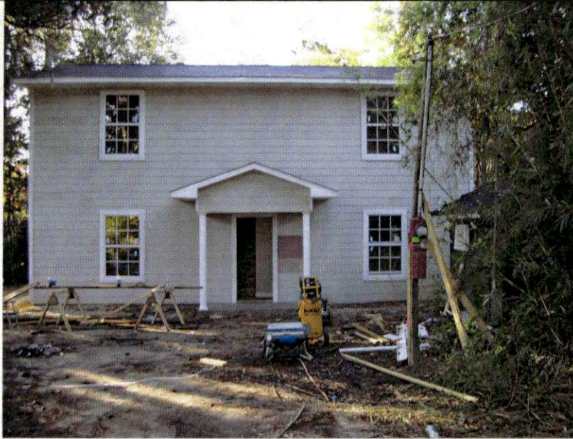
25 NOVEMBER 2008 -- FRONT VIEW
