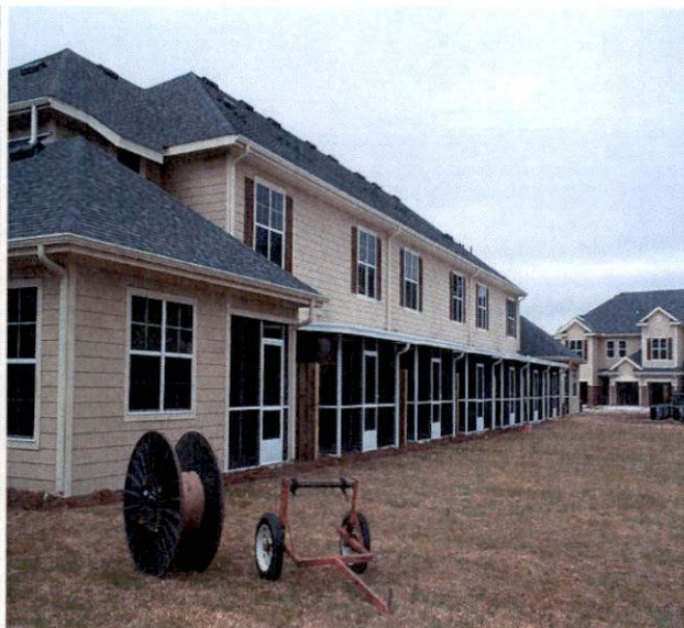
Bldg. 15 Rear view (taken 2/14/07)
