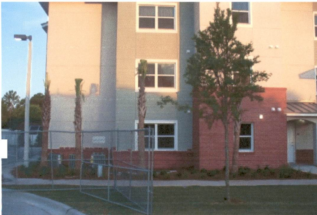
North End of Building
