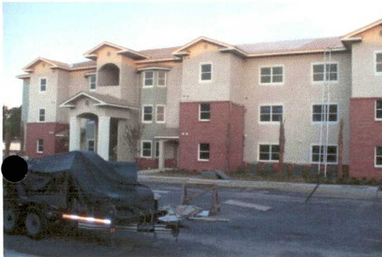
East side of Building - Center to South
