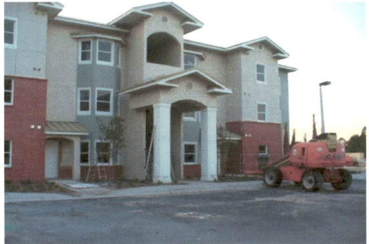
East side of Building - Center to North
