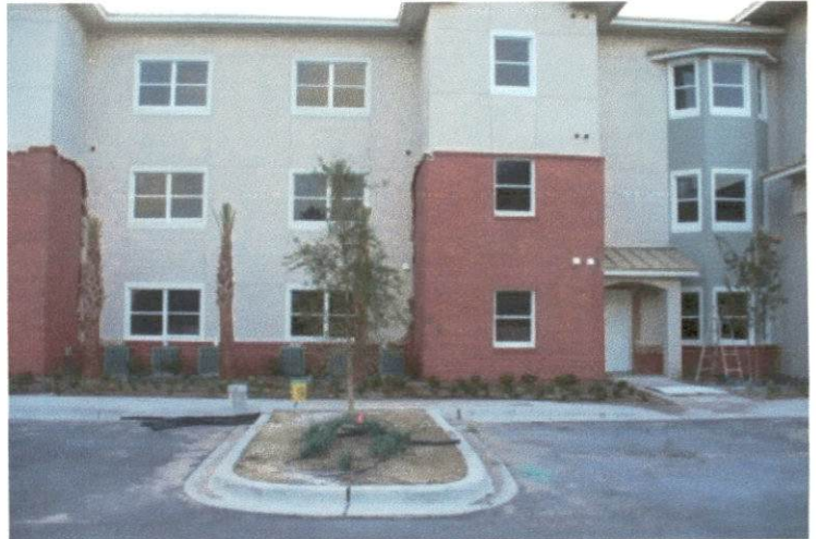
West Side - Center of Building with A/C Units
