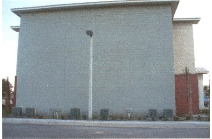
South end of Building
