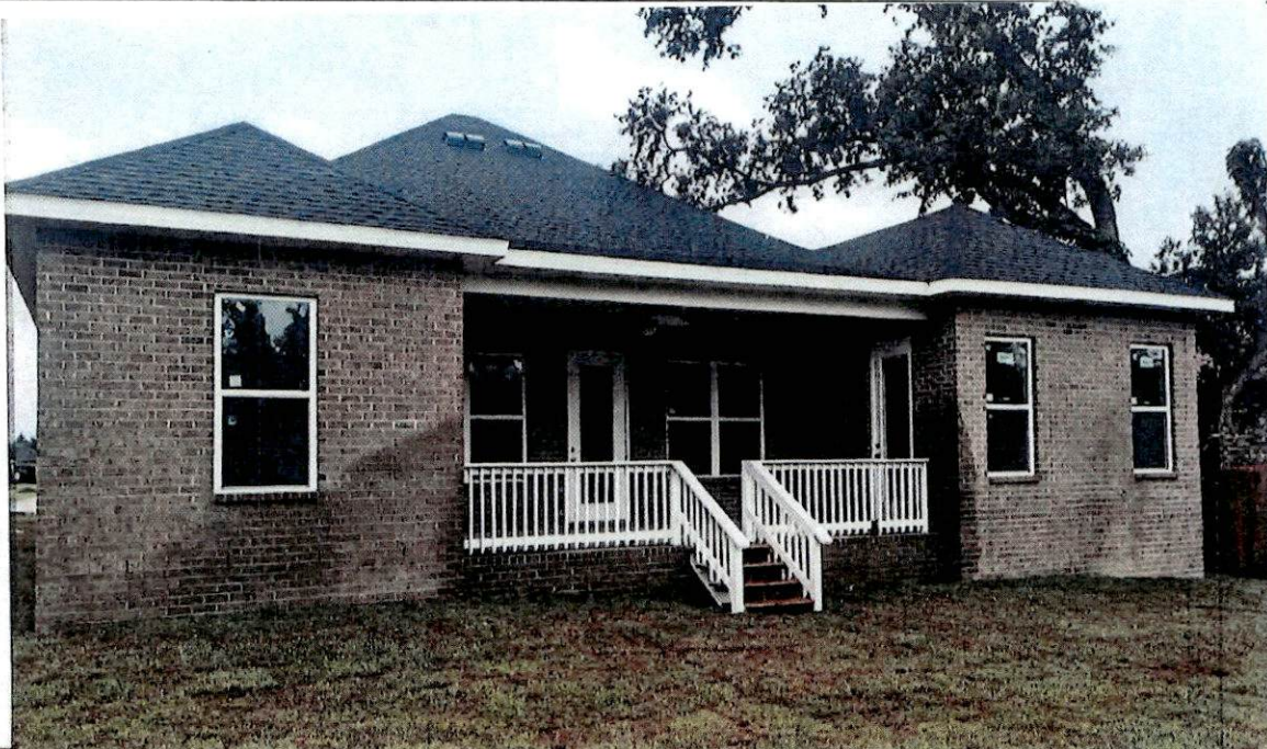
Photo Two Caption: REAR VIEW
